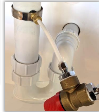
Drain clamp to PRV assembly
