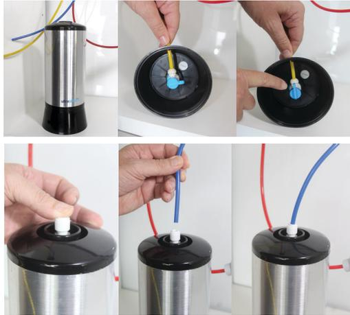
Note: You can cut the tubes to be shorter if you like, but we recommend leaving them long enough to pull the UltraStream unit out of the cupboard to change the filter.
